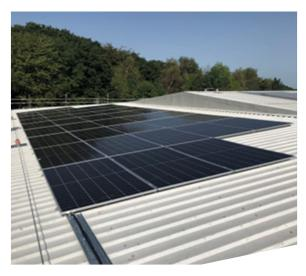
The scheme included the installation of rooftop solar photovoltaic panels in parallel with general roof fabric improvement and rooflight replacement, the latter providing for better insulation and natural lighting and thereby reducing future occupier energy demand for heating and artificial light.
